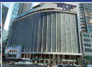
Insular Life Building Makati
