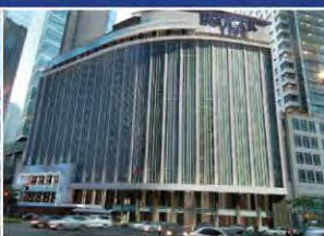
Insular Life Building Makati
